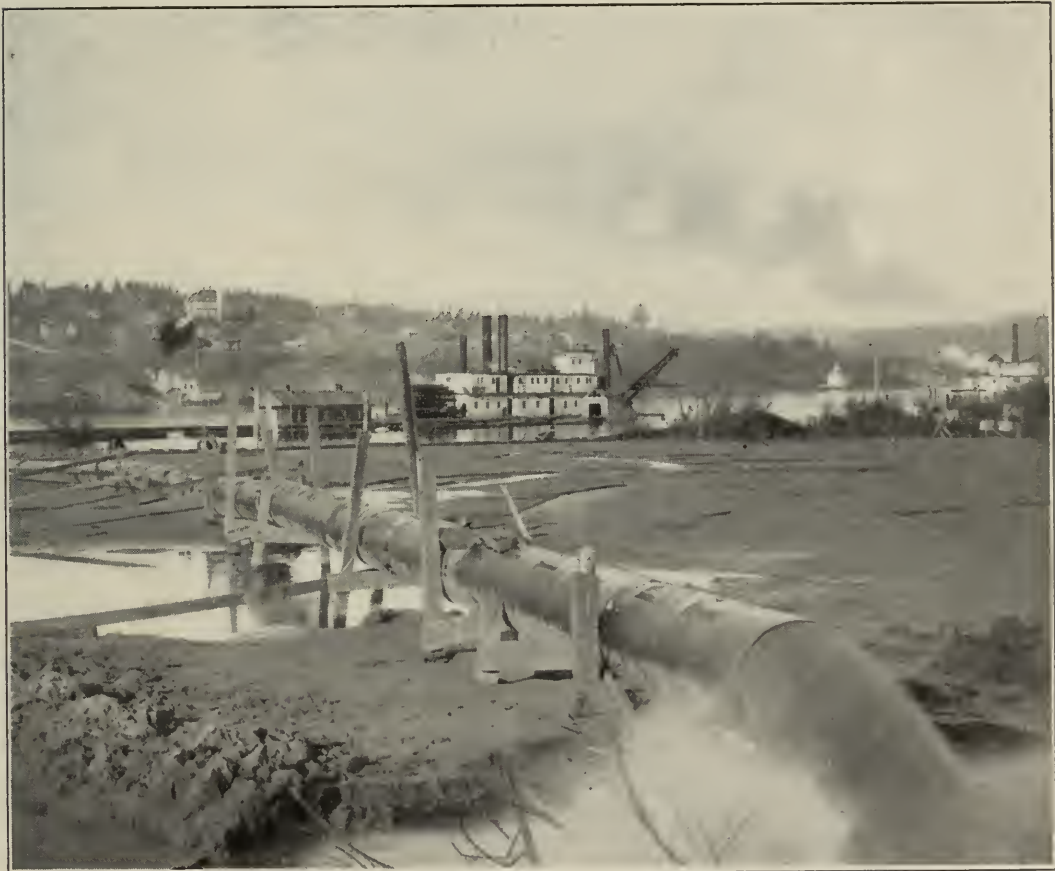
FIG. 33. SHORE DISCHARGE OF HYDRAULIC DREDGE KING EDWARD.
